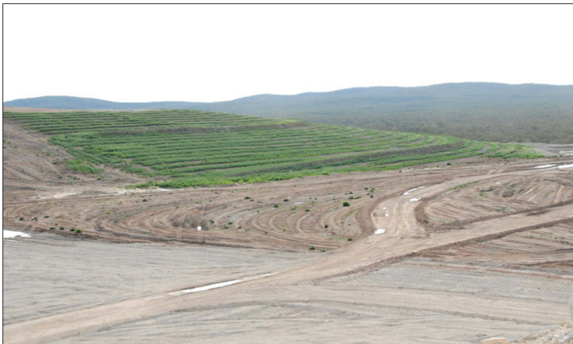
Plate 6-3 Tarrawonga Coal Mine - Northern Emplacement Reshaping and Cover Crop Establishment (2011)
